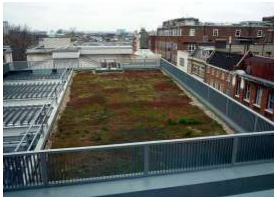
Green roofs are popping up on buildings throughout the district
